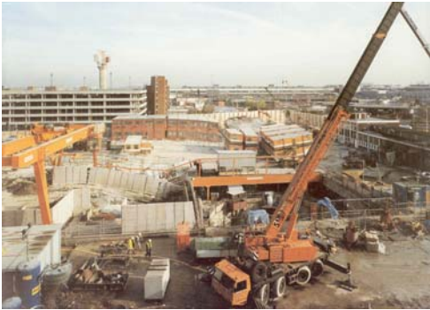
Fuel depot Shaft looking NE from Terminal 3 Car Park
